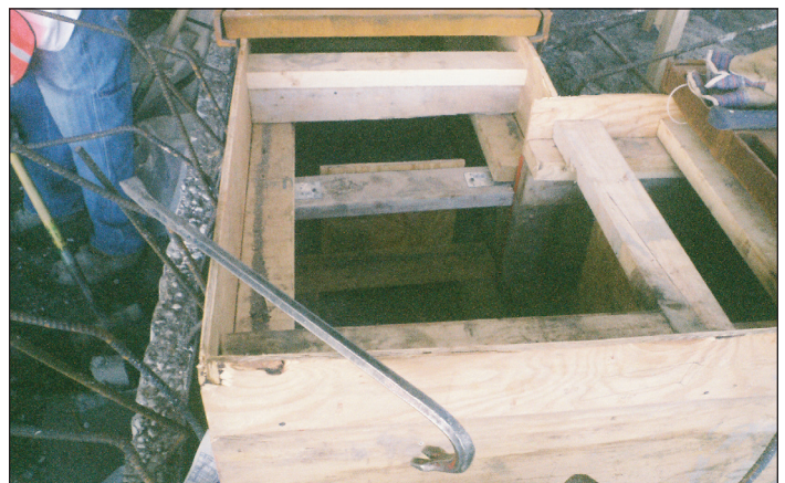
Z882 Install with Rebar Clips vs. Cast-In-Place Wood Forming.
