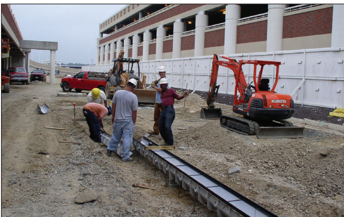
Z882 Install with Rebar Clips vs. Cast-In-Place Wood Forming.
